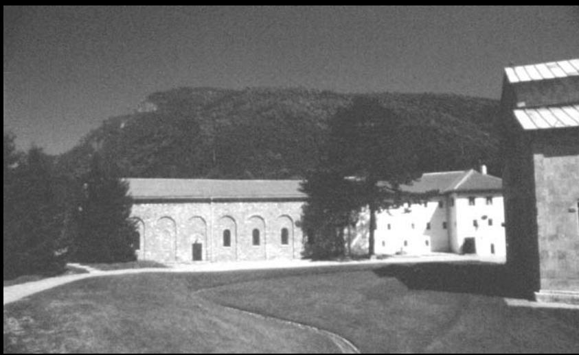
The refectory and the archimandry, view from the south
