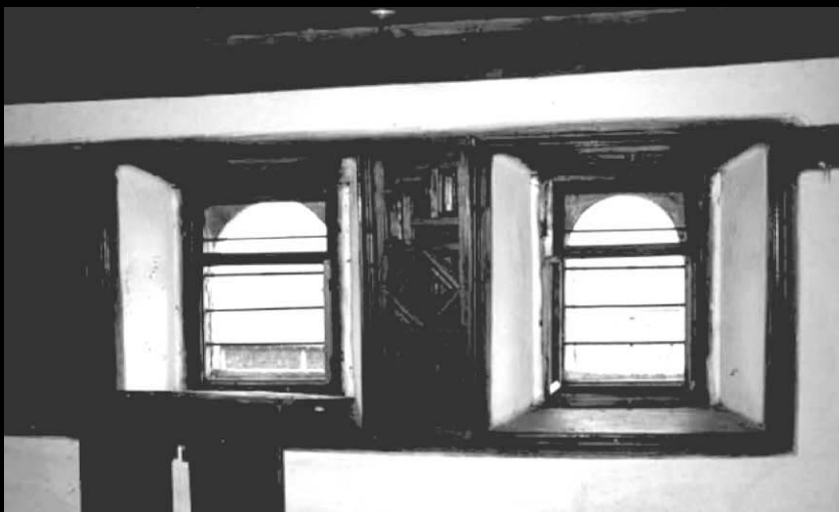
The interior of the guest room on the 2 nd floor
