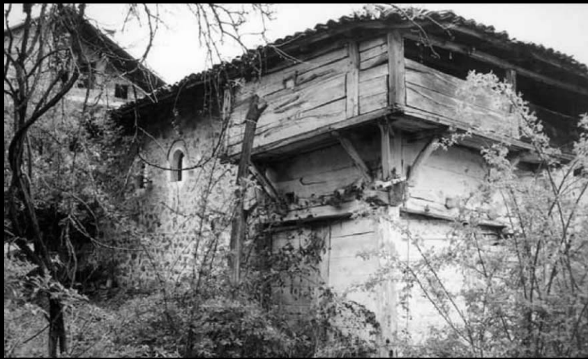
The southwestern corner of the timber terrace
