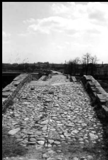
The condition of the cobble paving of the bridge
