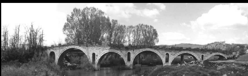
The view of the bridge in 2001
