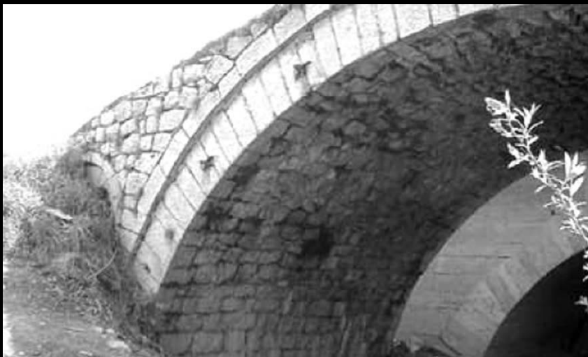
The arch of the old bridge
