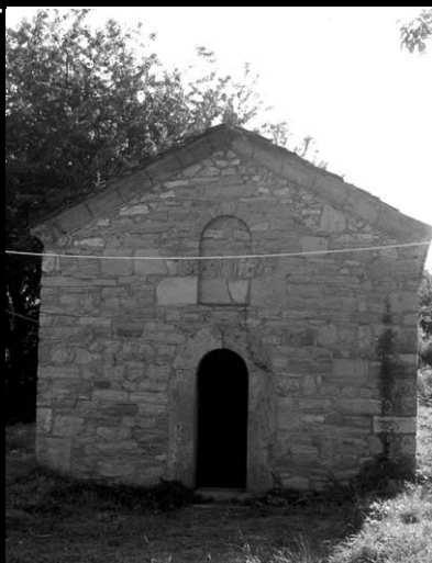
The west façade of the church
