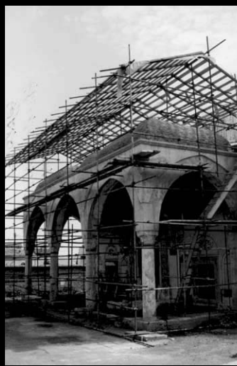
The portico and the minaret during restoration
