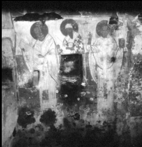
The south wall of the nave, frescoes after the fire
