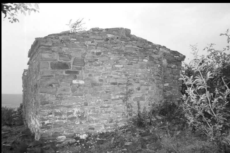
The eastern façade of the church with the altar apse
