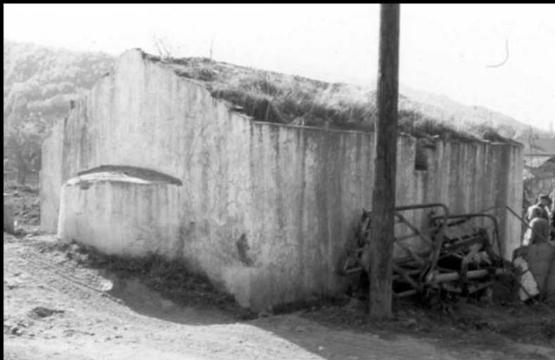
The roof and the apse after the removal of the roofing
