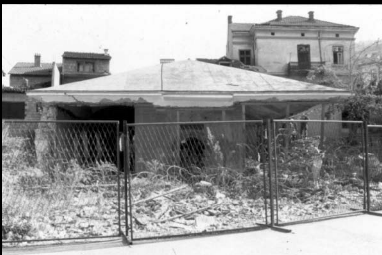
The church after the destruction, view from the west
