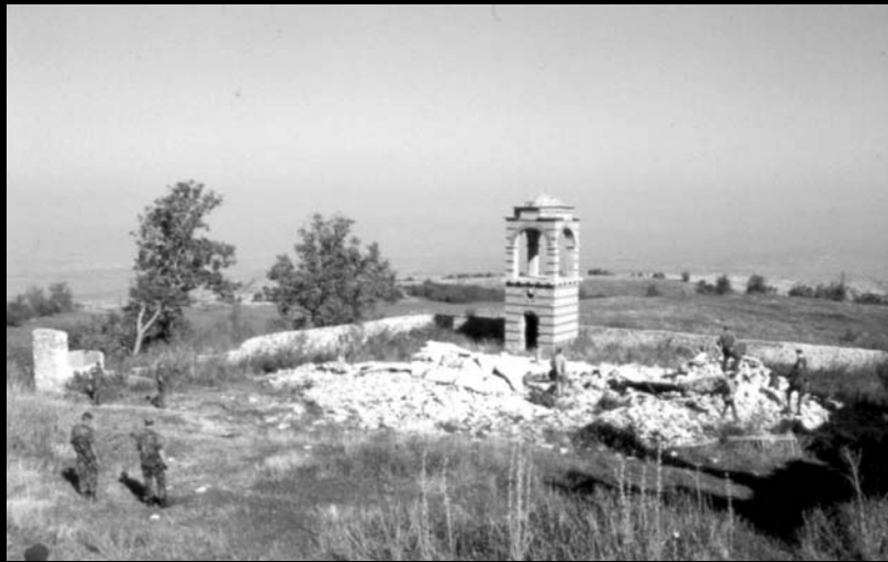
Remains of the church and the belfry after the destruction, view from the southeast
