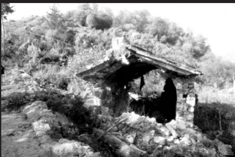
Ruins of the church with the remains of fresco decoration, view from the east
